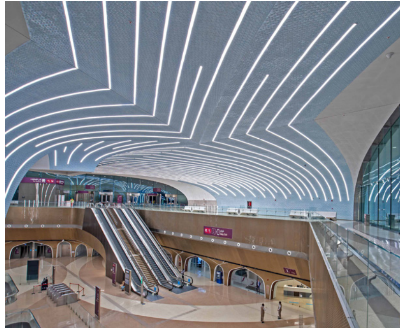
[19] Msheireb station – Central station of Doha Metro Network
