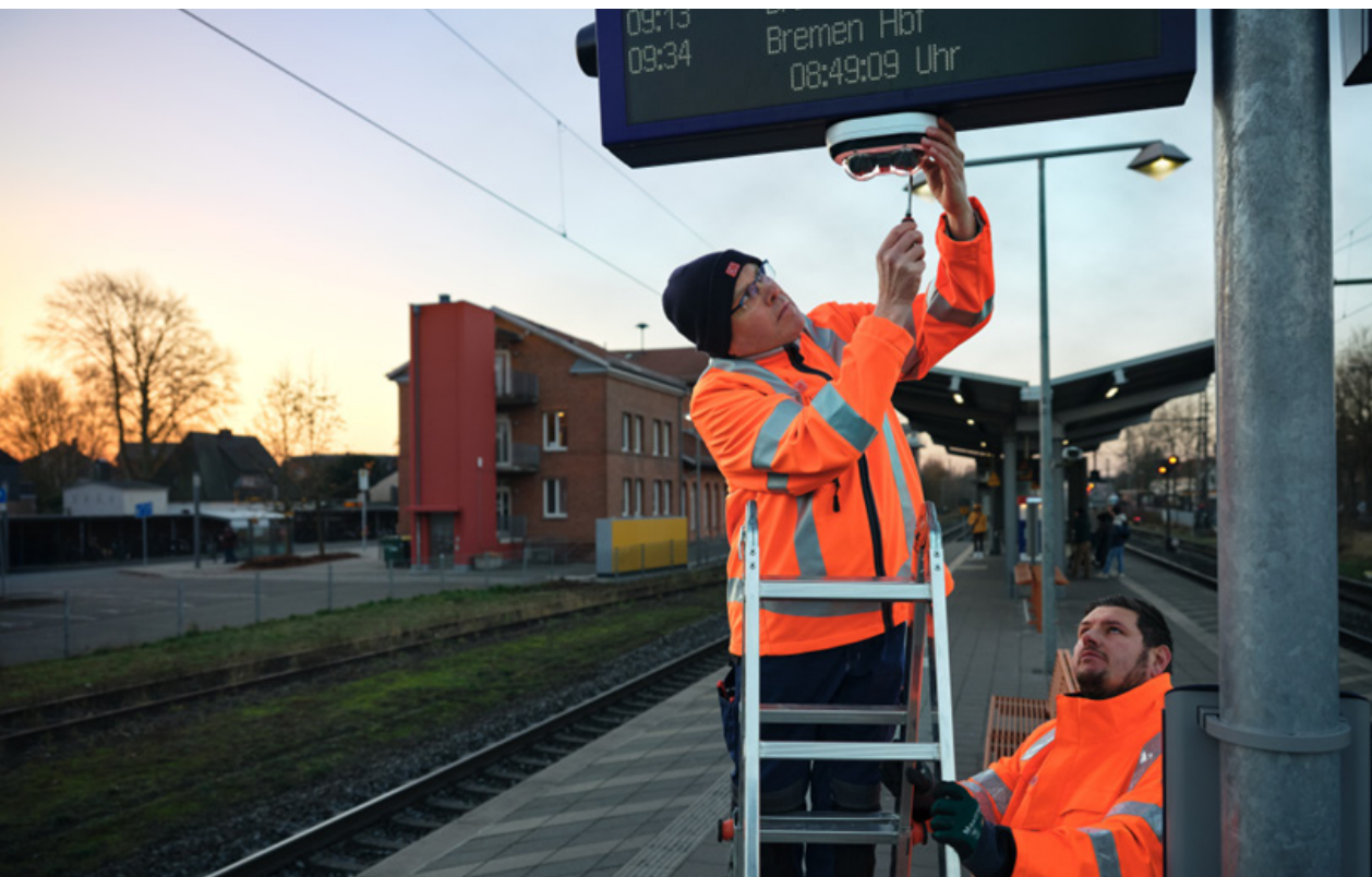
[3] DB InfraGO employees are installing a security camera on the platform
