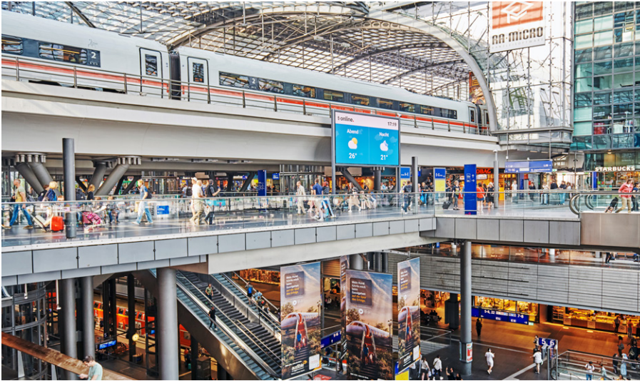
5: Metropolitan Hub Berliner Hauptbahnhof
